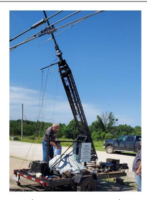
Charlie, WBØHWL and Jesse Jones, KDØETU working on putting up the crank-up tower with attached 40 meter dipole, G5RV, and triband Mosley TA-33 yagi.
